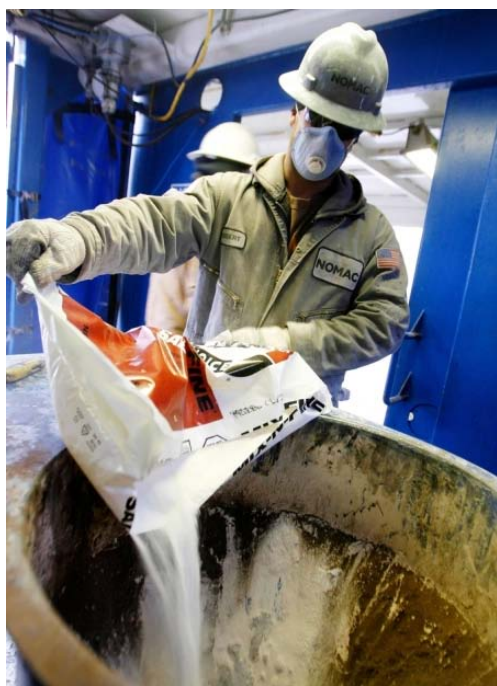
A worker pours salt into a mixer as he prepares drilling fluid - a combination of water, sand and chemicals - for fracking. Photograph by: TIM SHAFFER, REUTERS
